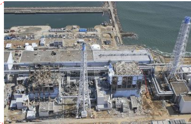
Fukushima #1 nuclear power plant
